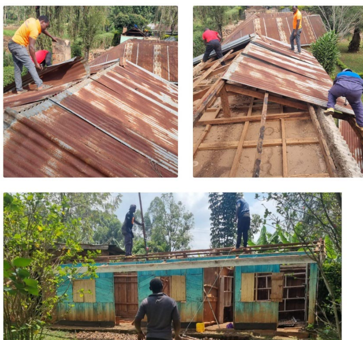
Removing of the old leaking iron sheets
